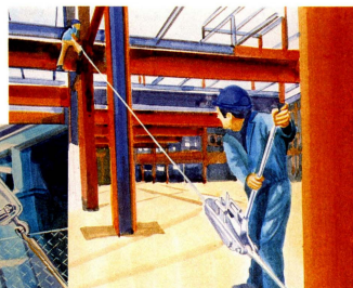
SUPER TIL used for steel alignment during erection.
